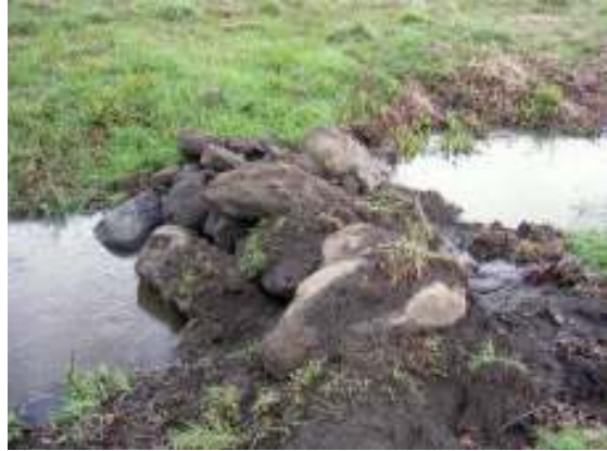
Using Rocks to build a rock dam
