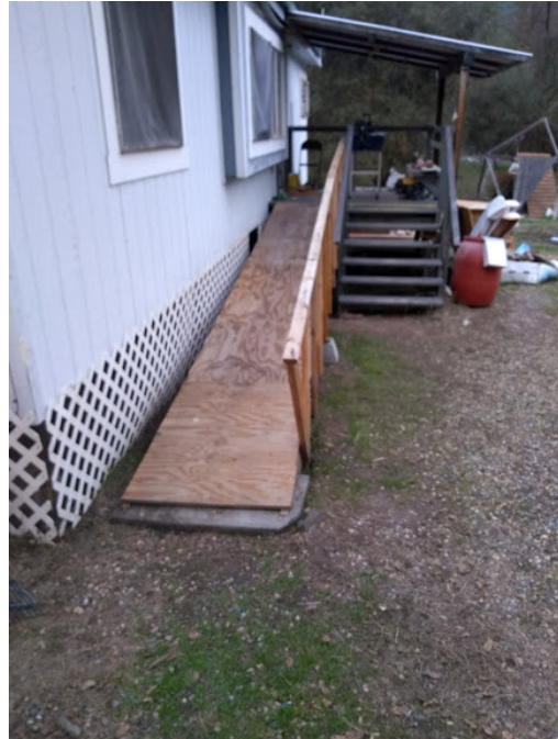
Added ramp access to home.
