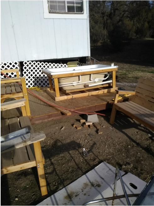
Putting a Jacuzzi Tub in at Cripple Creek resort (Tollhouse area)
