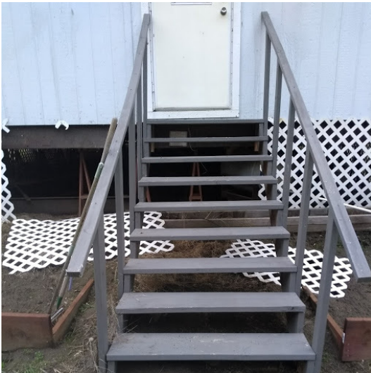
Replaced back porch and steps.
