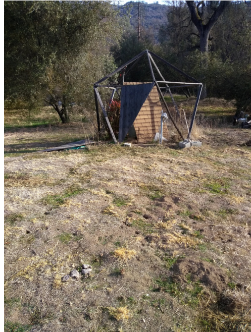
Old pumphouse will come down for dome structure (Have new pump)
